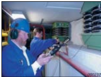
Fig. 3 Using FFT to troubleshoot vibration insulation in a large power plant
